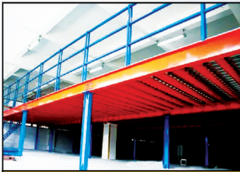
I BEAM MEZZANINE
